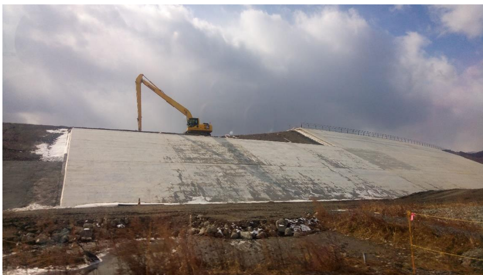
Sea wall is under construction.
